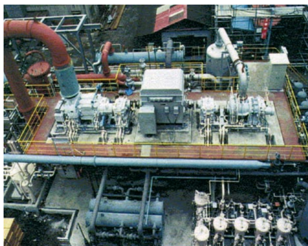
Figure 6. 'Wet and dry combination' for Ladle Gas Service in steel mill.
