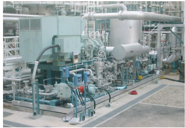
Figure 4. Hydrogen (90%) recycle gas for heavy catalytic cracked gasoline (HCCG) process.
